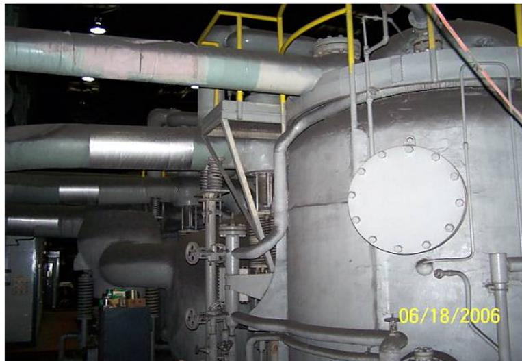
*Figure 6: Mercury Vapor Lines and Mercury Condenser Boiler*
