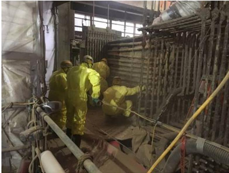
**Figure 11: Unit 2 Removal of Boiler Tubes**
