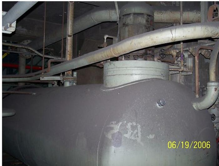
*Figure 5: Liquid Mercury Storage Tank.*
