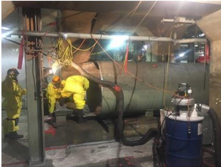
***Figure 14: Removal of Mercury Storage Tank Through Non-Thermal Cutting***
